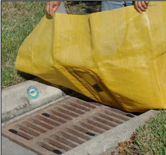
**Step 2:** Place the unrolled GrateGuard Plus over the grate and align the center open bermed area (Overflow Opening) of the GrateGuard Plus so that it is over grate openings. The open bermed area (it should be facing up) is the emergency overflow port in case there is flooding in the street. In some cases this means offsetting the opening from the center of the grate to place it over the openings in the grate.
