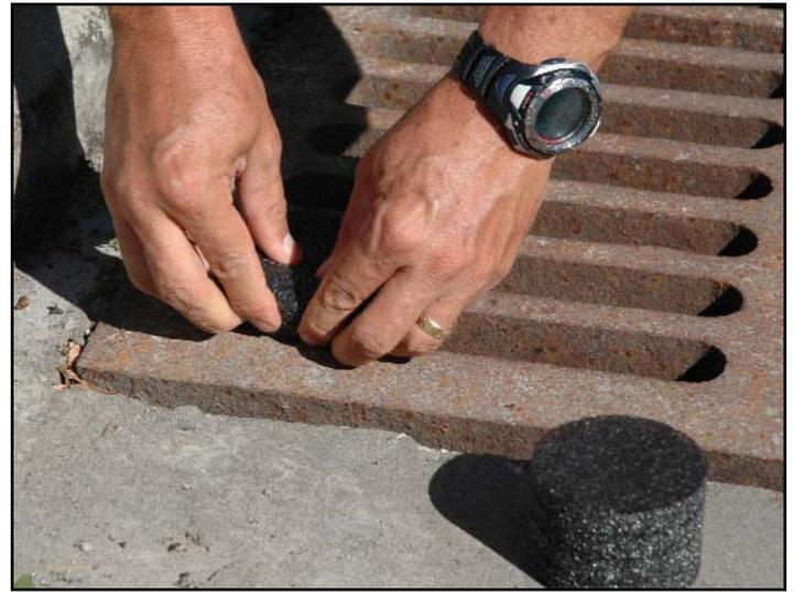
**Step 1:** Insert the foam Holding Blocks into each corner of the grate and place two of the blocks into the outside center of the grate along the longest side. Insert them so they are flush with the grate. You should now have 6 Holding Blocks inserted around the perimeter of the grate.
