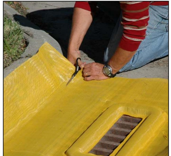
**Step 3:** Once it is positioned, cut the excess material on the sides of the GrateGuard Plus, so that it will cover the grate or is slightly larger. Do not cut it undersize. Leave it properly positioned so it is covering the grate.
