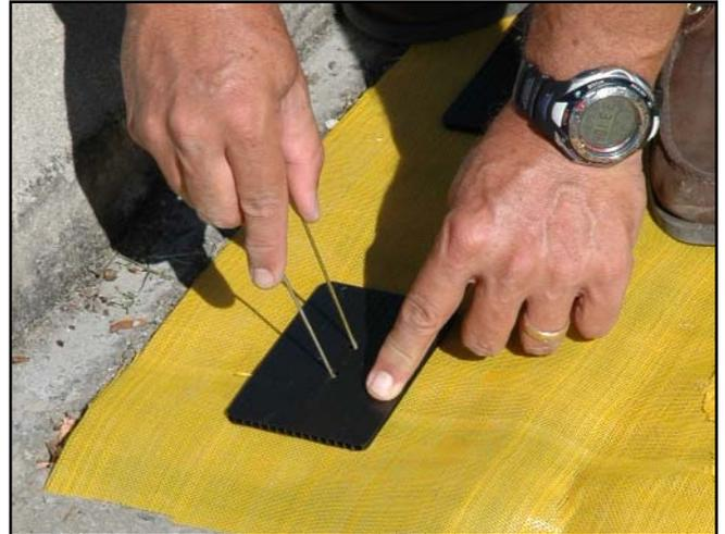
**Step 6:** Repeat Step 5 for each of the other five Holding Pads and Holding Blocks. **Note:** Be sure to pull the fabric tight in both directions before you insert the U-Pin into the next Holding Pad and Block. This will insure the best fit to the grate.
