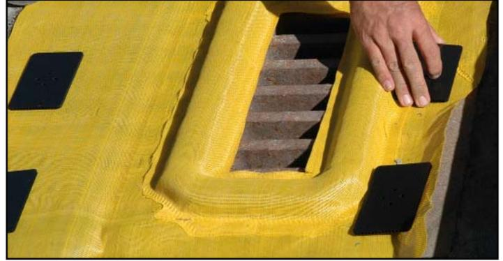
**Step 5:** Insert one of the U-Pins through two of the holes in the center of the Holding Pad, through the yellow fabric of the GrateGuard Plus and keep inserting it down into the Holding Block in the grate until the U-Pin is flush on the Holding Pad.
